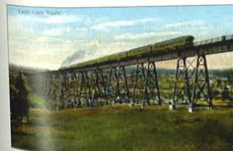
▲ The Latah Creek Trestle.
