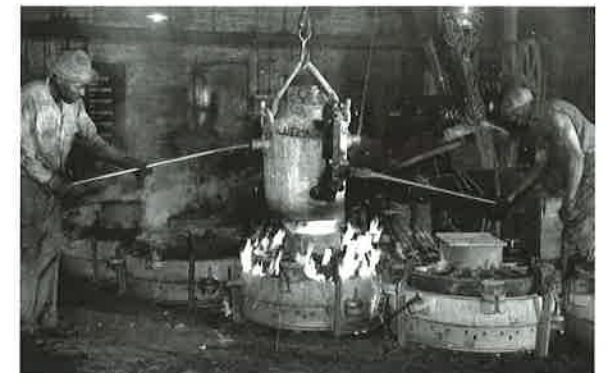
▲ Steel workers at the Griffen Wheel Company in Tacoma.
