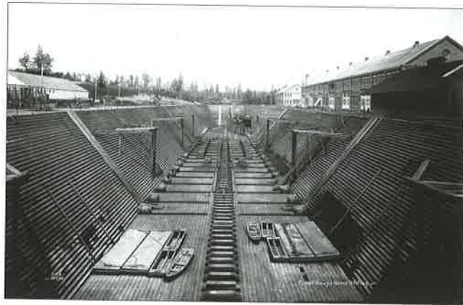
▲ Shipbuilding became a major industry in Washington during World War II. This photograph is a wooden drydock at Bremerton's Naval Shipyard during World War II.
