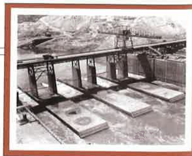
▲ Diversion channel to redirect the Columbia River for construction.
