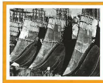
▲ Construction of Bonneville Dam's spillways.
