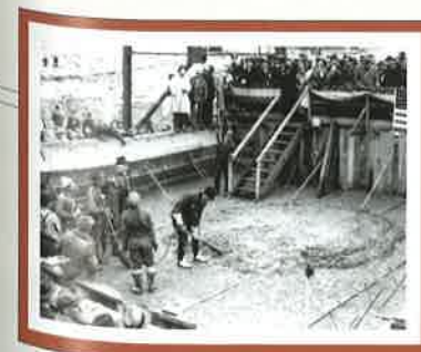
▲ The first concrete load of the Grand Coulee Dam construction.
