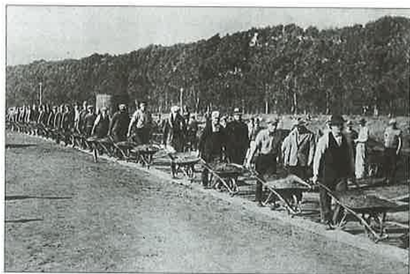
▲ Members of the Civilian Works Administration (CWA) construct a road in Washington in 1934.
