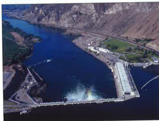
▲ Rocky Reach Dam
