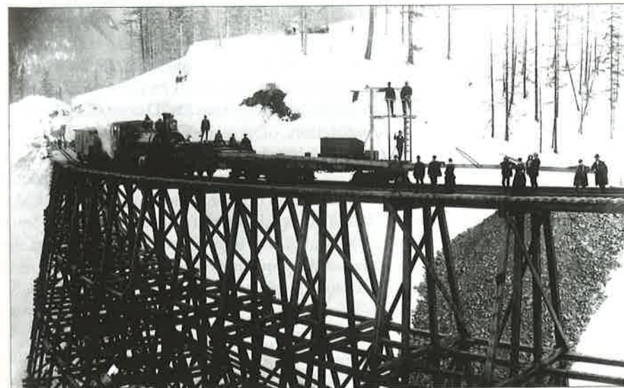
▲ Construction of the Mosquito Creek Railroad.
