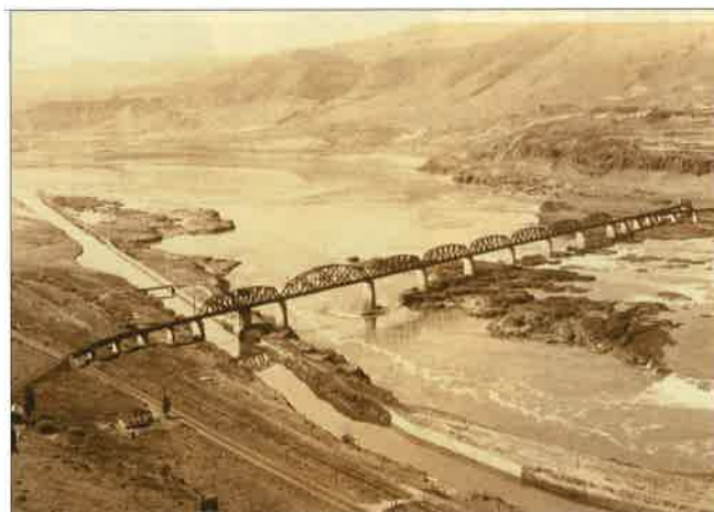
▲ Columbia River Railroad Bridge at Celilo Falls.
